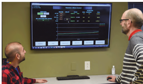
Sam Tatulli, left, biosolids mechanic, and Nick Menninga, general manager, adjust the Landia GasMix equipment via the SCADA system.
