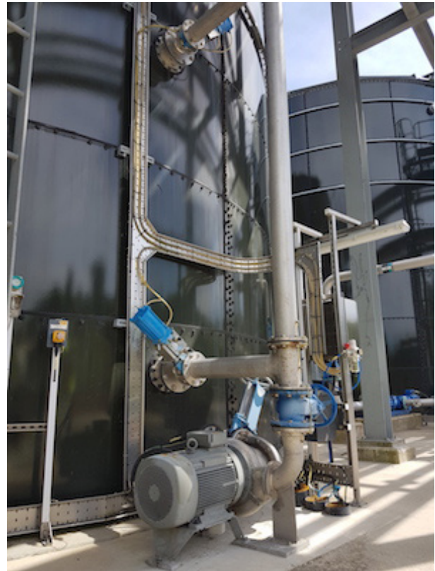
The sewer treatment plant in Jersey, the largest of the Channel Islands between England and France, requested the equipment be installed at ground level rather than raised platforms.
